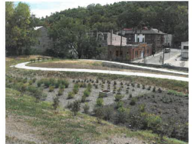
St. Francis Bioinfiltration Basin during Dry Conditions
