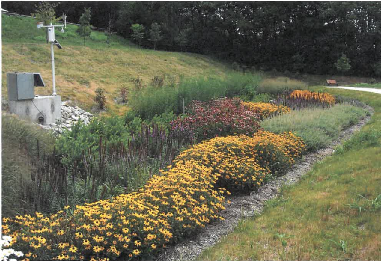
St. Francis Bioinfiltration Basin (2011)
