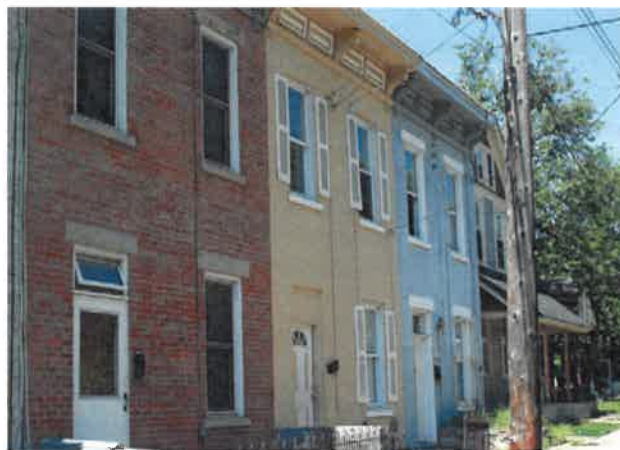
Existing Small Scale Residences in the Lick Run Watershed
