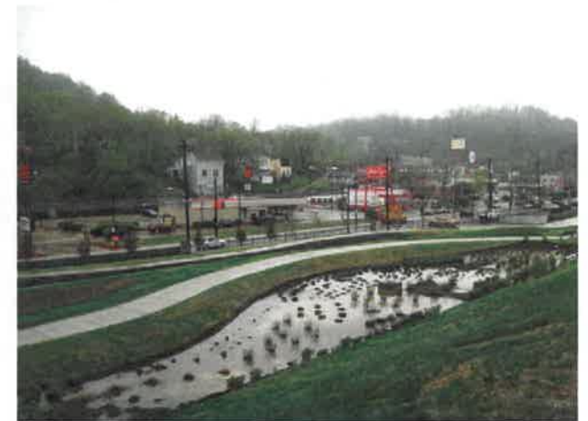
St. Francis Bioinfiltration Basin during a Rain Event
