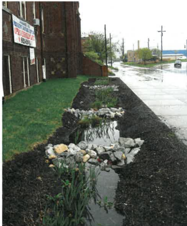
Bioinfiltration Basin at Immanuel United Church
