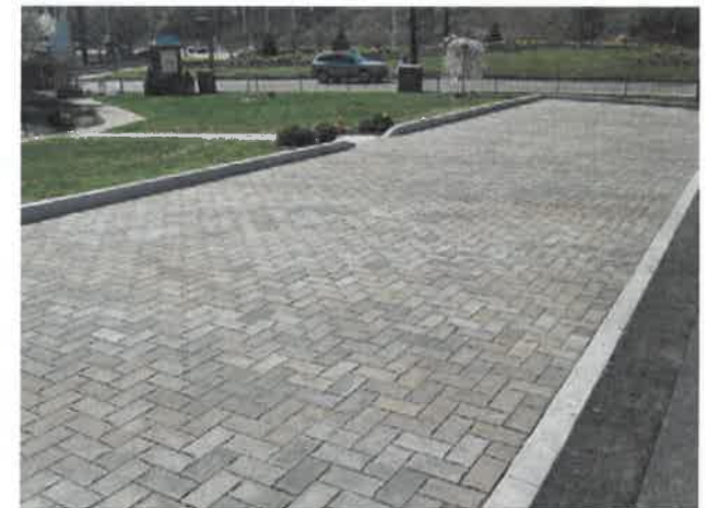
San Antonio Site After Installation of Permeable Pavers
