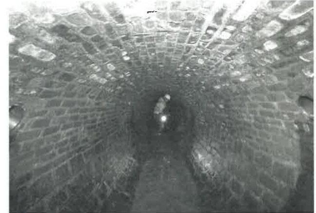
Brick sewer from the 1800s
